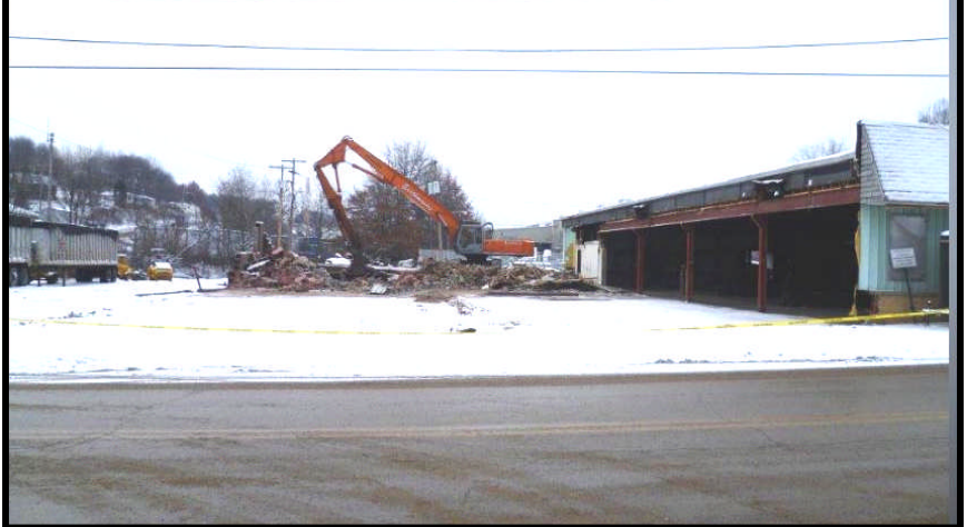
Future Home of the Petrolia Volunteer Fire Department
